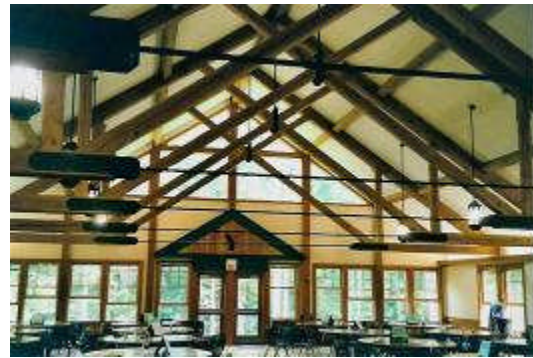
Acoustic tile highlights the beautiful trusses at YMCA Camp Takoda, NH
